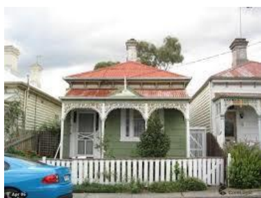
A view of 7 Falmouth St, taken prior to recent alterations. (Credit: onthehouse.com.au)
